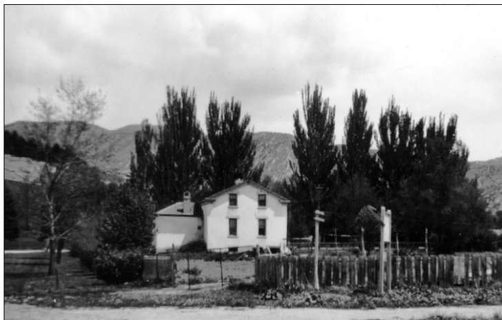
The house in Manti where Winnie lived after the fire
